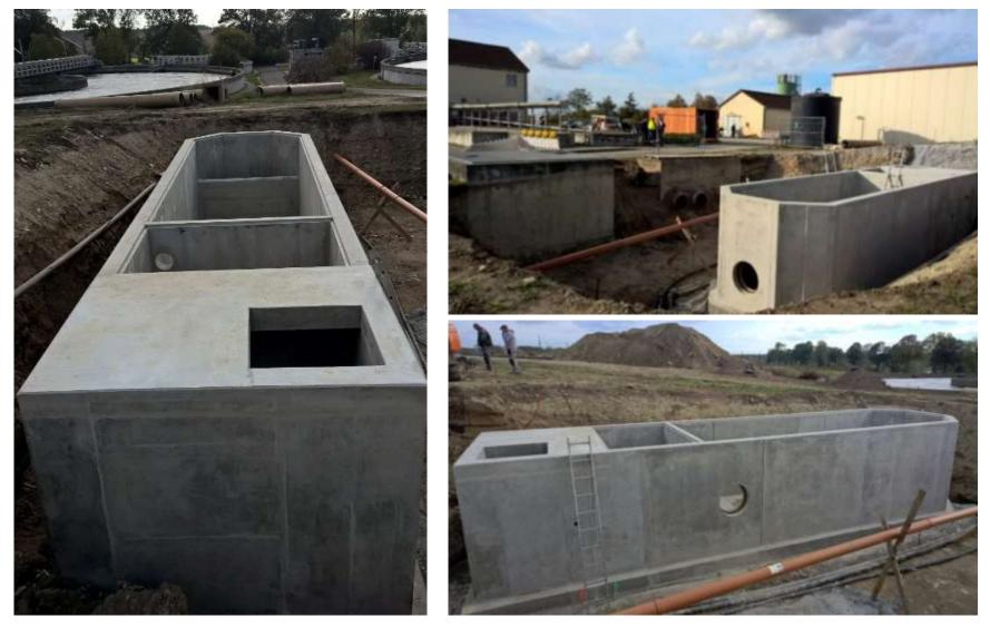
Civil works for flow bypassing to the Drum Screen LIQUID
